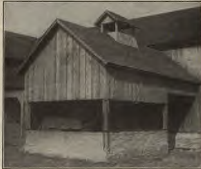
FIG. 235. — Covered manure shed with cemented bottom.
